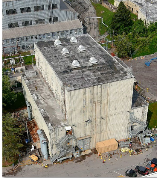
Deactivation and demolition of 3042
