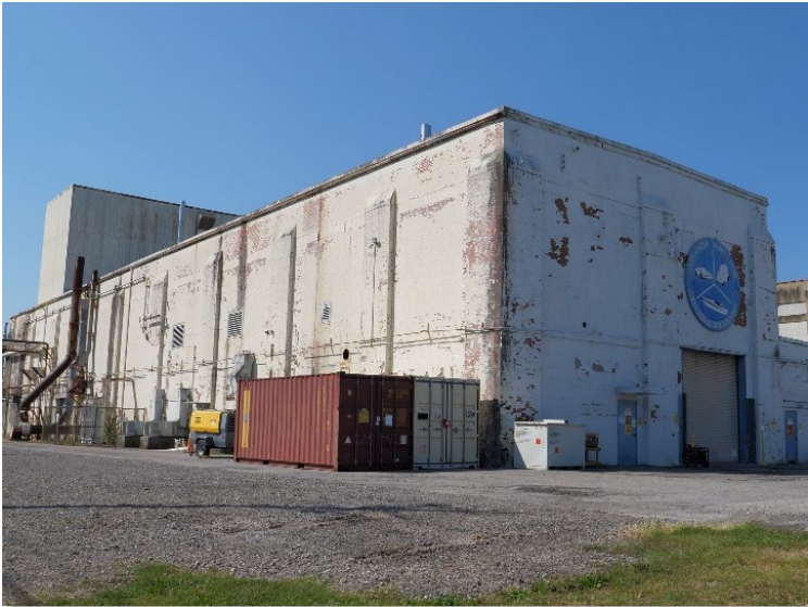
Old Steam Plant demolition
